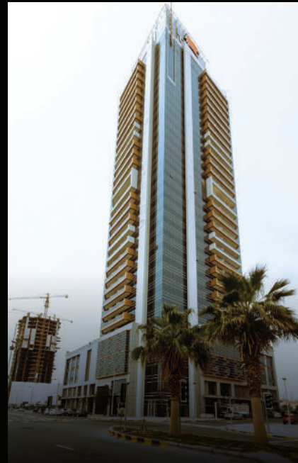
Al Manarah Tower JVT Dubai
