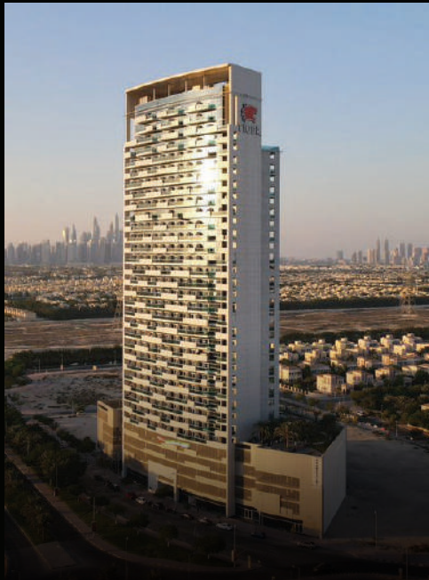
Al Jawahara Tower JVT, Dubai
