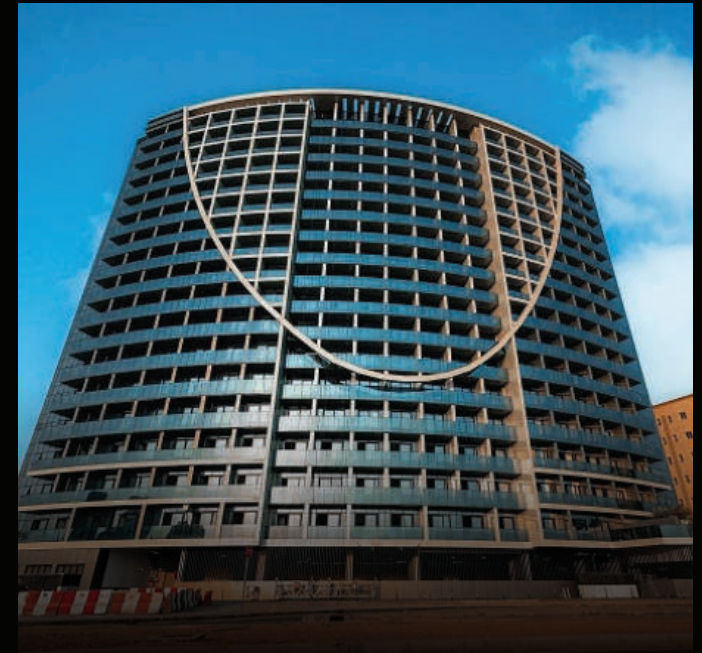
The V Tower Dubai Land
